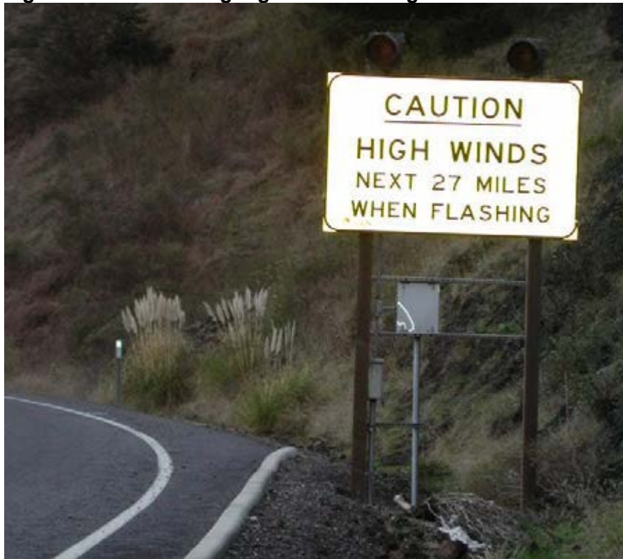
Figure 3. Wind Warning Sign with Flashing Beacons
