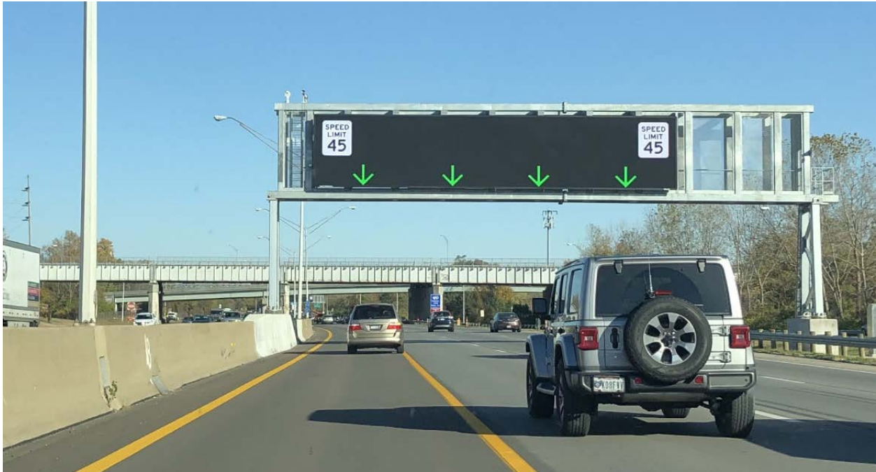
Figure 5. SmartLane Active Traffic Management Example Source: Ohio DOT.
