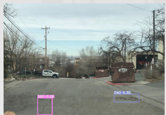
Pavement Condition Assessment
