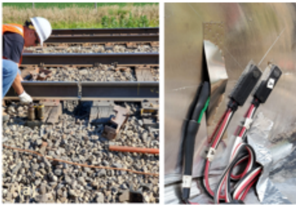
Rail destressing & instrumentation
