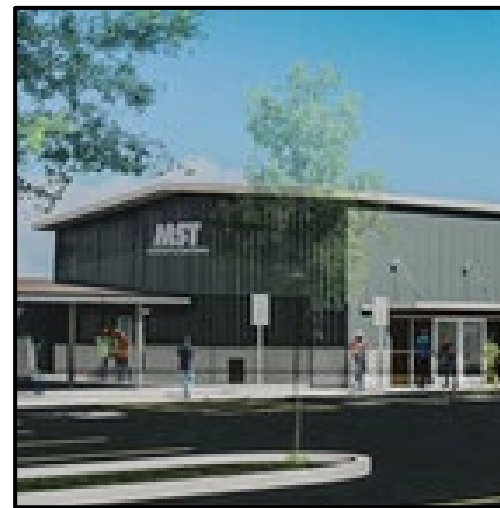
MST O&M Facility Monterey-Salinas, CA
